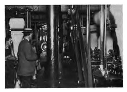
Narrow Aisles between Machines with Unguarded Belts and Pulleys.
